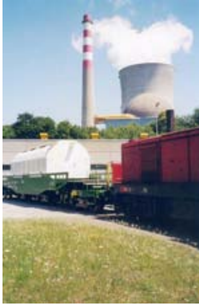
FIG. 17. Departure of spent fuel on a wagon from a nuclear power plant to be reprocessed at the La Hague facility.
